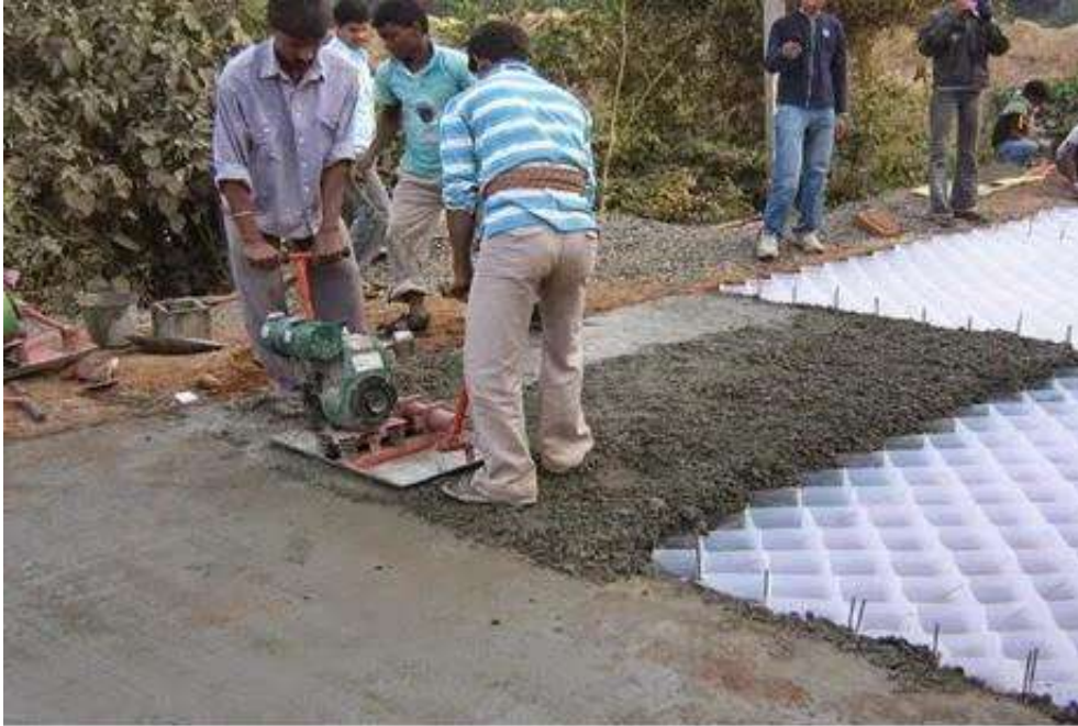
Figure 3: Laying of Cell filled Concrete Pavement.
