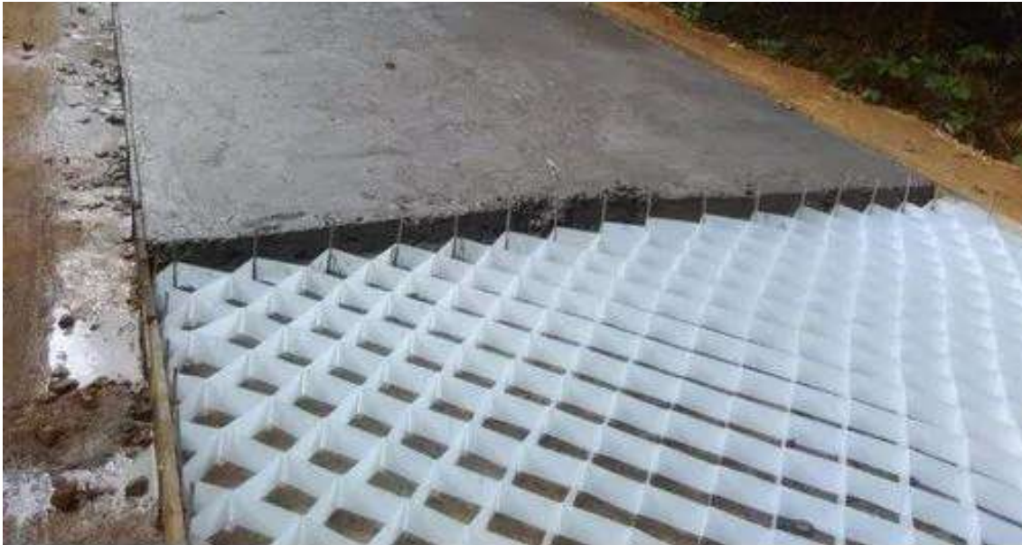
Figure 1: Cell Filled Concrete Pavement.
